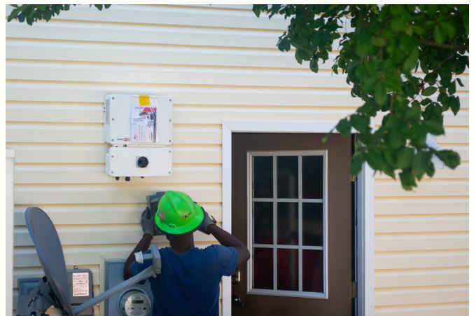
Extern working on the installation of solar panel inverter.
